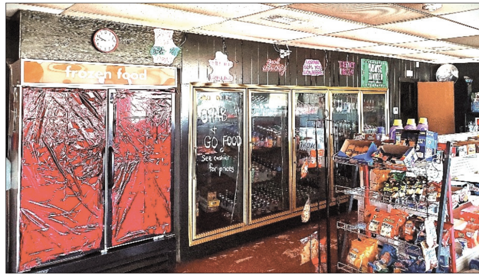
Interior freezer, coolers, and shelving.
