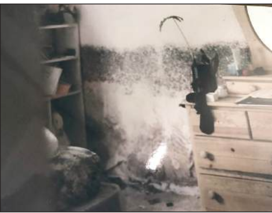
Destruction after Katrina hit
