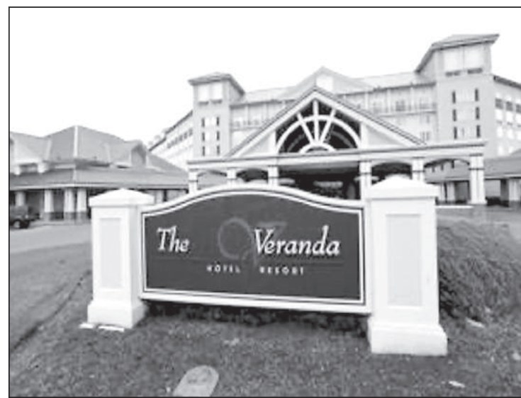
The Veranda hotel on May 13, 2014, in Tunica Resorts, Miss., is one of two hotels being considered to house unaccompanied immigrant children in northwest Mississippi. The hotels were part of a Harrah's casino complex that closed in 2014. AP PHOTO/ROGELIO V. SOLIS, FILE
