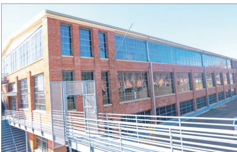
Mississippi Center for Innovation and Technology (MCITY) in Downtown Vicksburg
