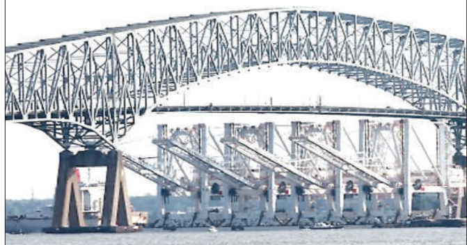
A portion of the Francis Scott Key Bridge in Baltimore collapsed after a large boat collided with it early Tuesday morning, and multiple vehicles fell. Photo and video, 11Alive Baltimore
