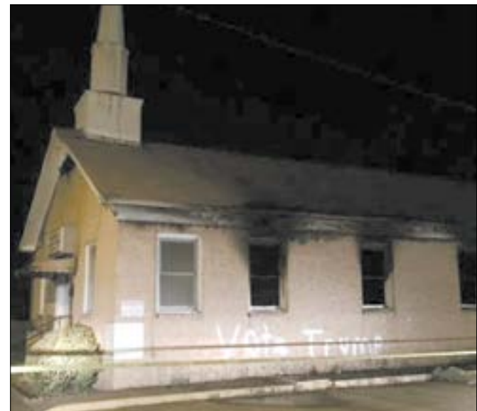
This is what remains of Hopewell M.B. Church in Greenville after a fire Nov. 1. PHOTO COURTESY GOFUNDME.COM
